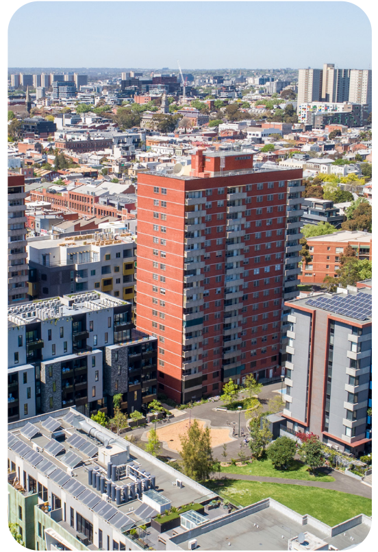
Carlton's old red brick towers will make way for more and better homes.
